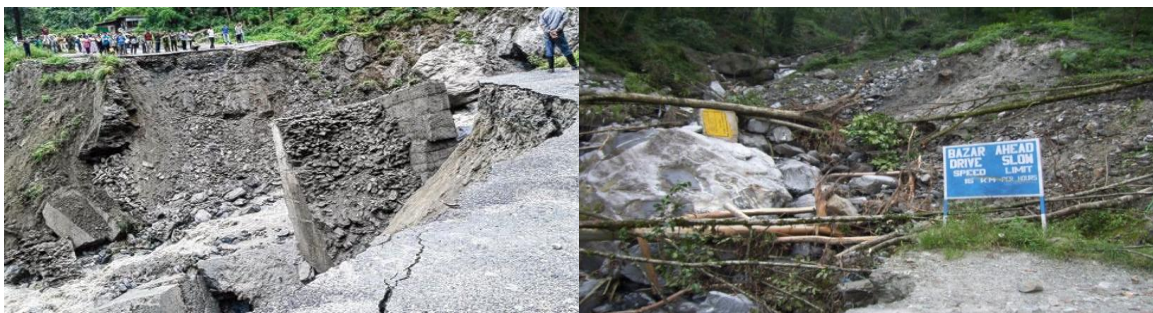
Photo Plate 6: Raffong Khola along Mangan Landslide
